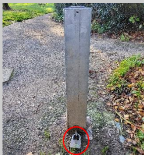
Figure 5 – Drop post padlock
